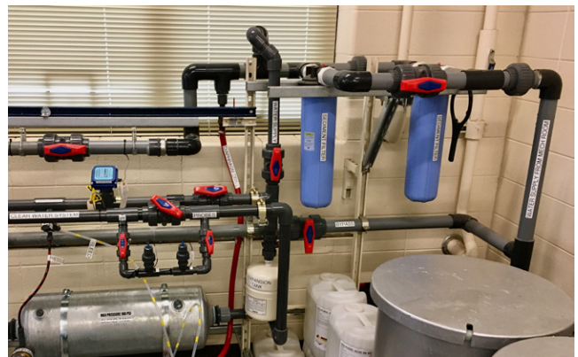
Figure 20. Sediment cartridge filters in blue colored casings, upper right.
