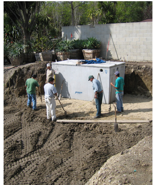
Figure 31. Slow sand filter schematic and during construction.
