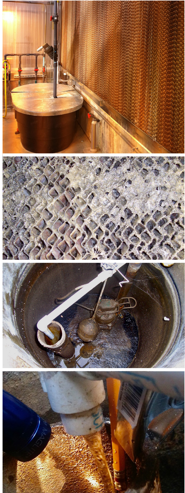
Figure 17. From top: evaporative cooling pad and reservoir; scale and biofilm accumulation on a pad; empty reservoir showing PVC-pipe bleed-off feeding into a drain pipe, close up of the bleed-off flow following adjustment.
