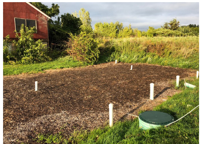
Figure 30. Woodchip bioreactor. 91
