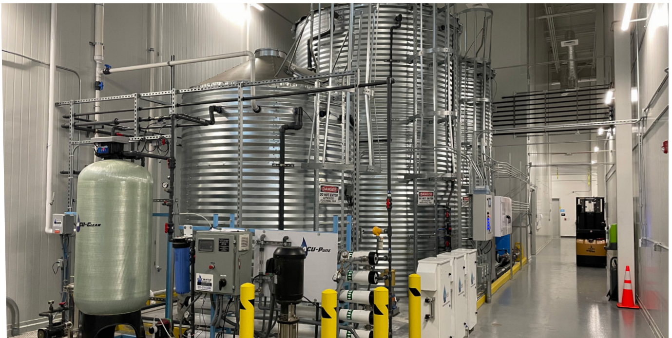
Figure 42. Water technical area at an indoor farm.
