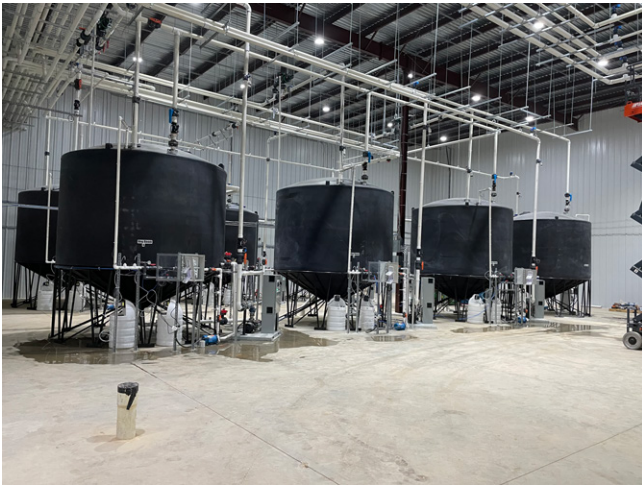
Figure 40. Rendering of nutrient dosing system with acidification and ozone disinfection. Nutrient dosing systems, day tanks, and associated plumbing.
